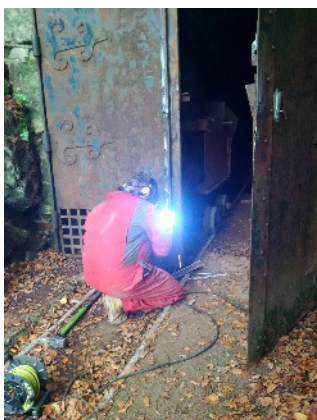
Welding some angle onto the outside of the door
