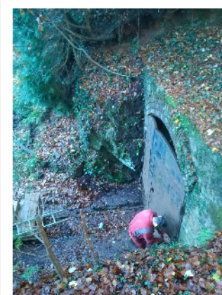
Cleaning up the mine door with a wire wheel
