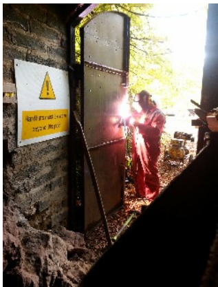
Welding a lock plate inside the mine door
