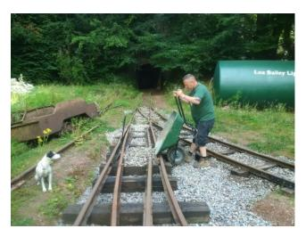
Since the May open days the main work at Lea Bailey has been ballasting the new track to the container and preparing to lay a new siding down to where the Eimco 24 resides beyond the lorry ramp beside the container.
