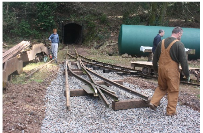
Laying out rails for new points
