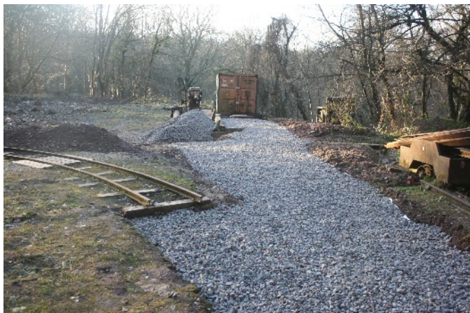
Spreading clean ballast ready for track laying
