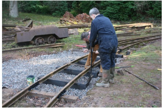
New sleepers and ballast on curve
