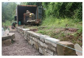
The retaining wall being built alongside the track to the container is nearly up to track level. It just needs a row of bricks laying on top. Then it should be ready for backfilling and then the track can be relaid - with sleepers and ballast!
