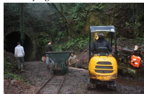
clearing mud at Drybrook end
