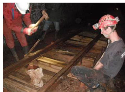
track laying in the tunnel
